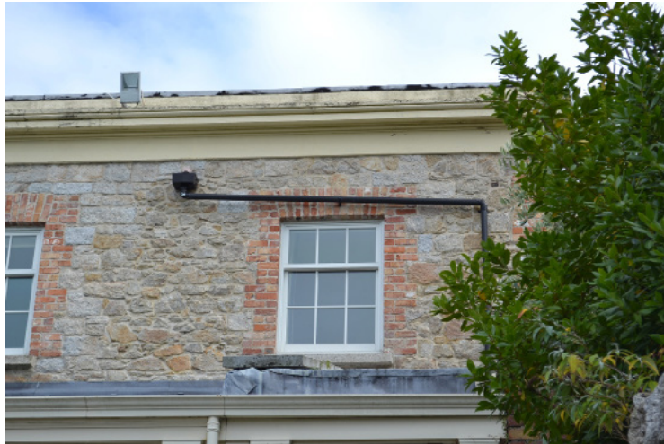
Detail of rainwater downpipe on western elevation.
