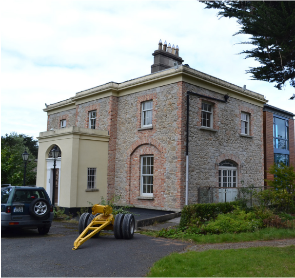
Cedar Mount - Current view from the south-east.
