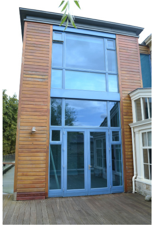
View of western elevation of rear extension.
