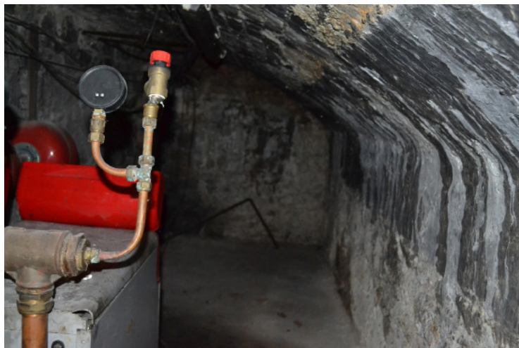
View of service space 02 looking east.
