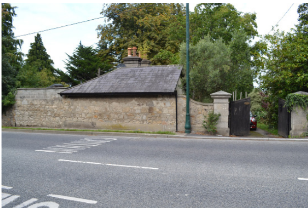
View of Gate Lodge (West).
