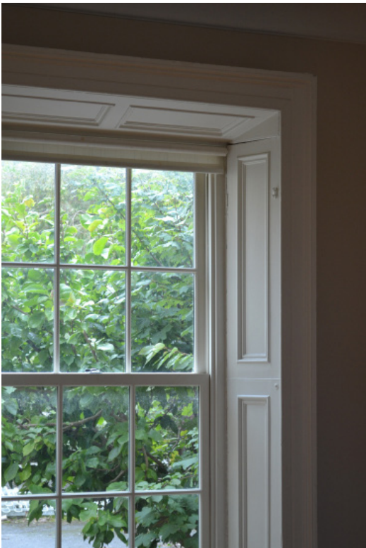
Detail of kitchen window.
