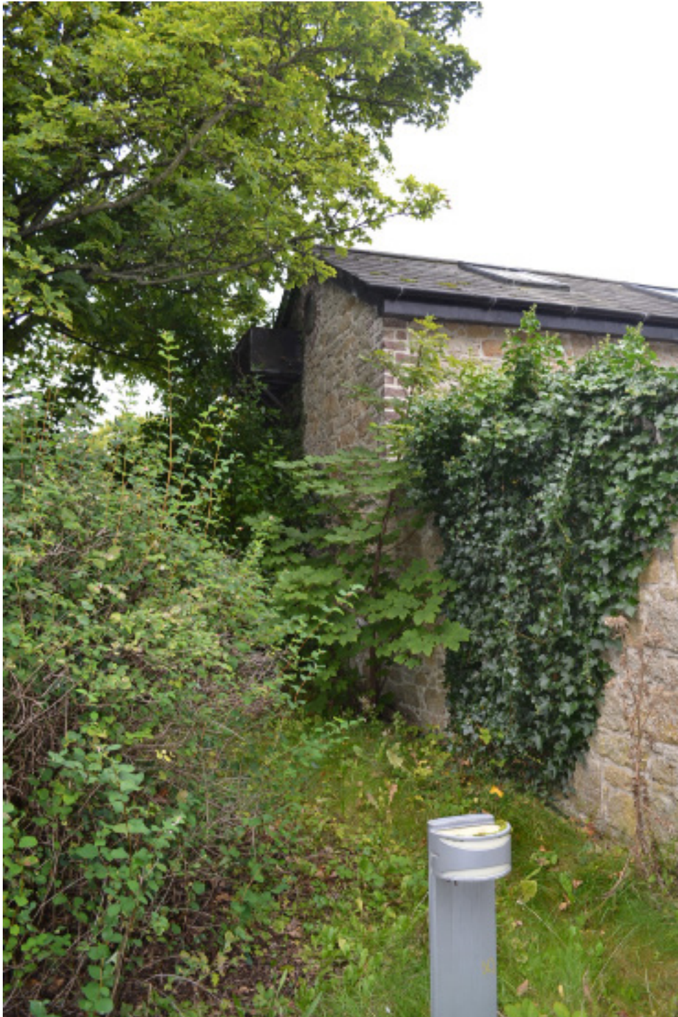
View of South Elevation.
