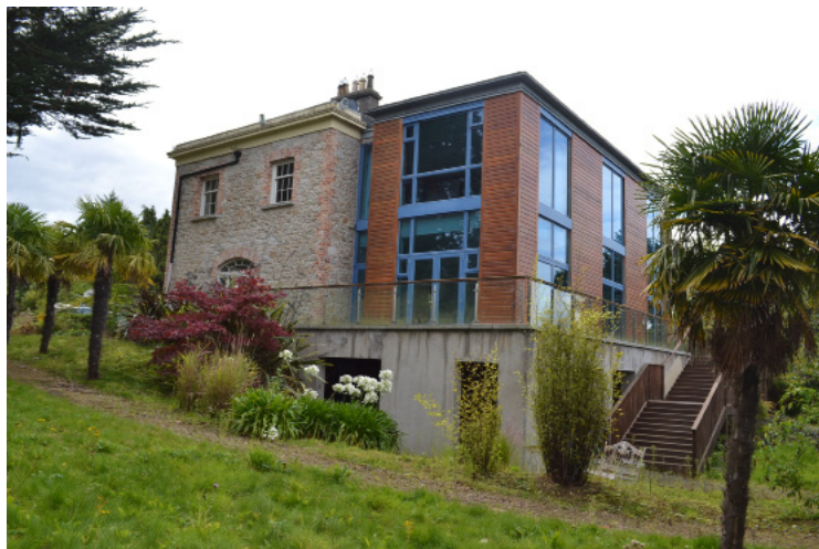
View from north-east.
