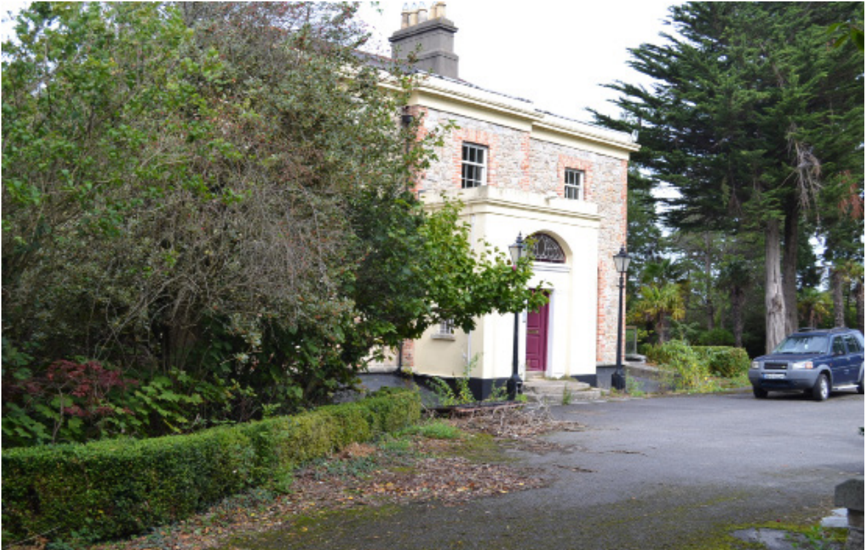
View form south-west.
