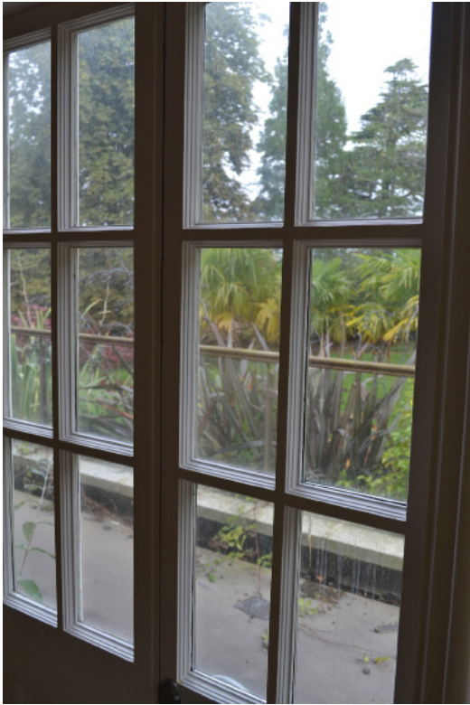
Detail of living room external door:
