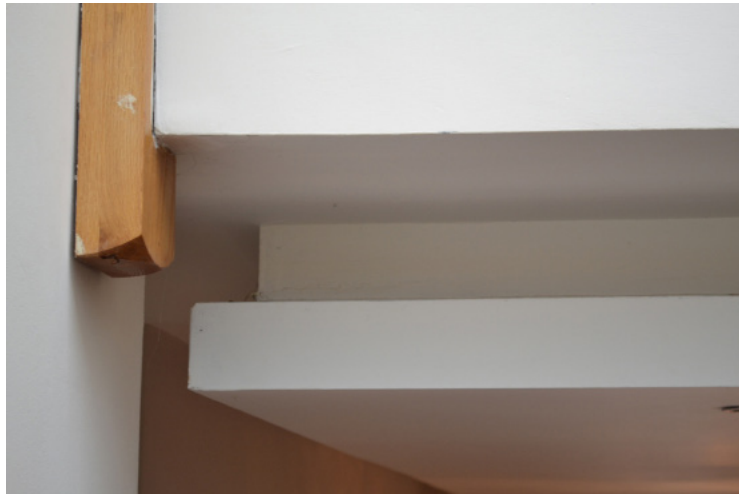
Detail of ceiling recess.
