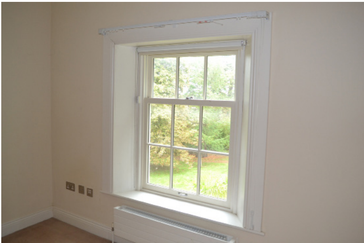
View of window in bedroom 01.
