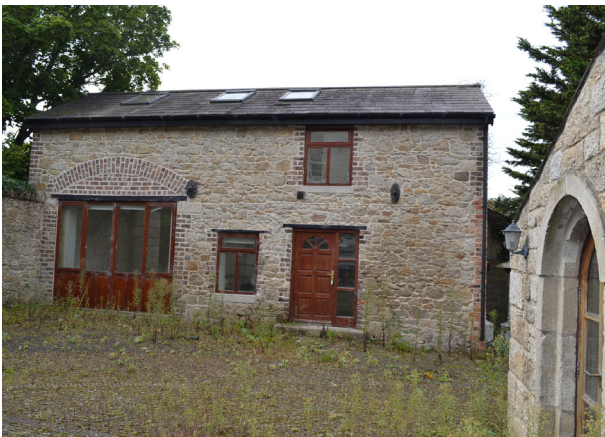
Coach House - current front (East) elevation.
