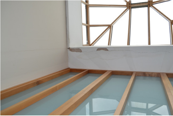
Detail of roof-light.
