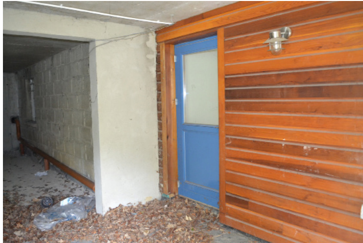
Detail of eastern section of loggia.
