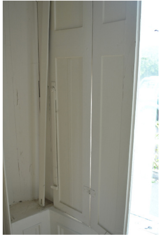
Detail of living room window shutter.
