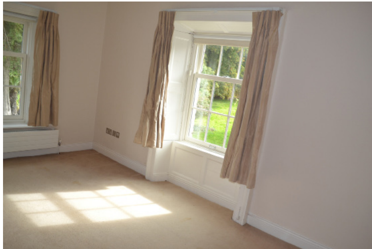
View of window in bedroom 02.
