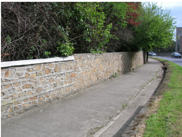
View of cement pointing to wall.
