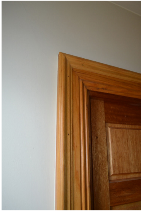
Detail of typical architrave.
