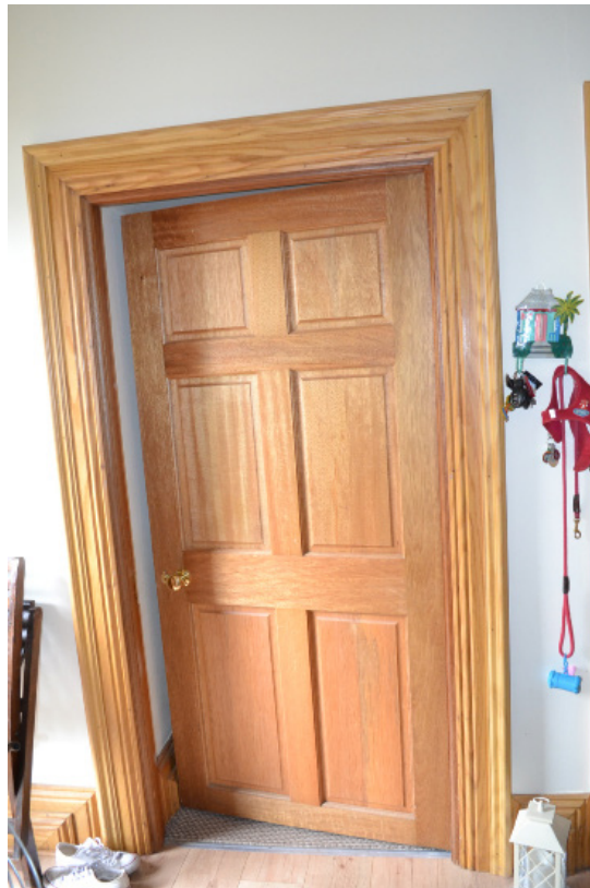
Detail of typical interior door:
