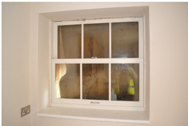
Utility room kitchen.
