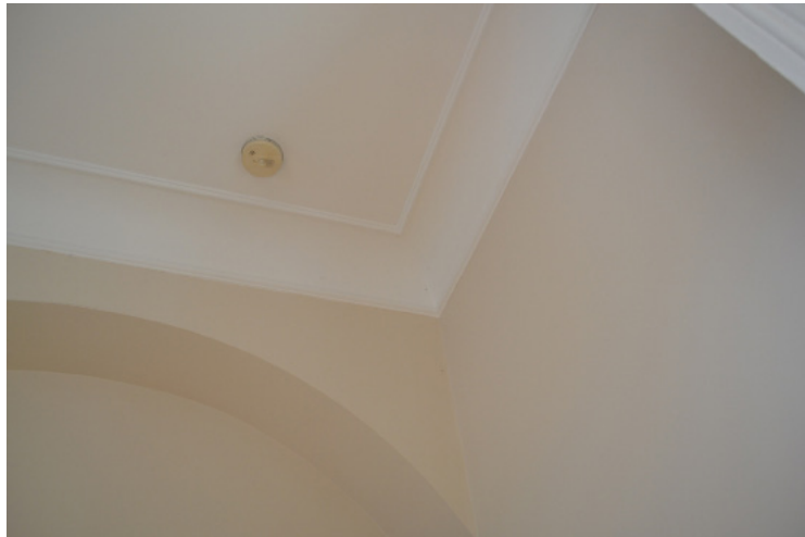
Detail of kitchen ceiling cornice.
