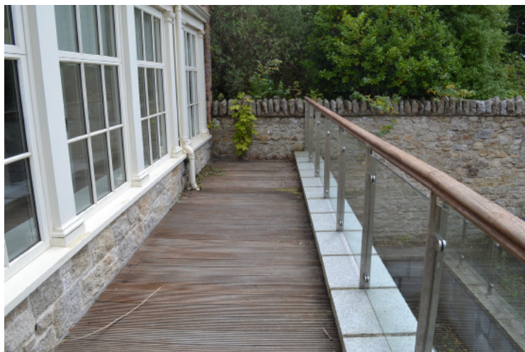
View of western section of terrace looking to the north.
