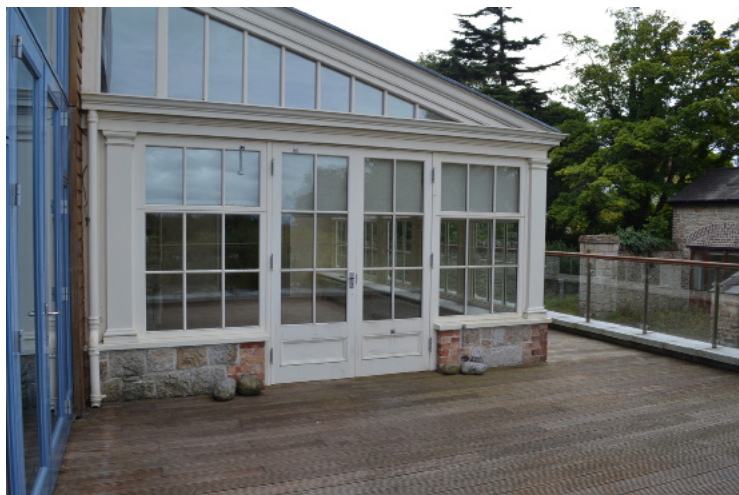
View of North Elevation of conservatory.
