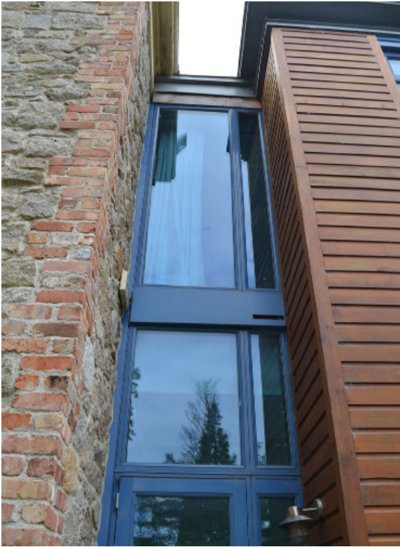
Junction between house and extension on east elevation.
