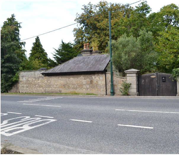
Knockrabo Gate Lodge (West) - current view from the south.
