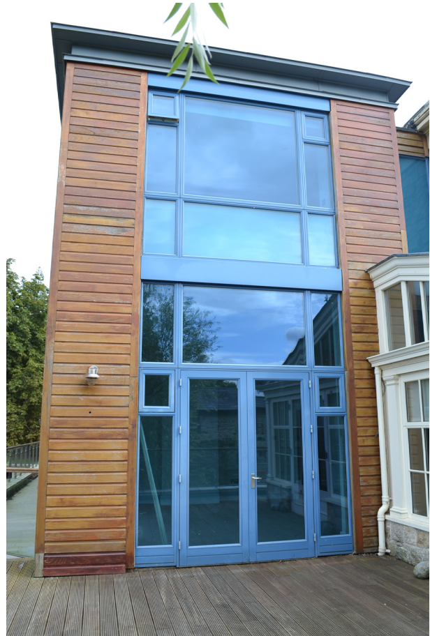
Cedar Mount - Current View of rear extension from the left.
