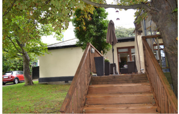
External timber stairs.
