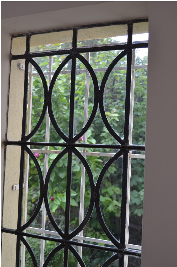
Cedar Mount - Entrance lobby window detail.
