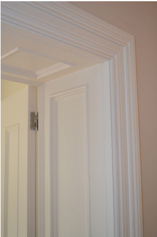
Detail of living room internal door architrave.
