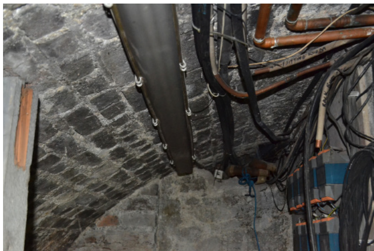
View of service space 02 looking west.
