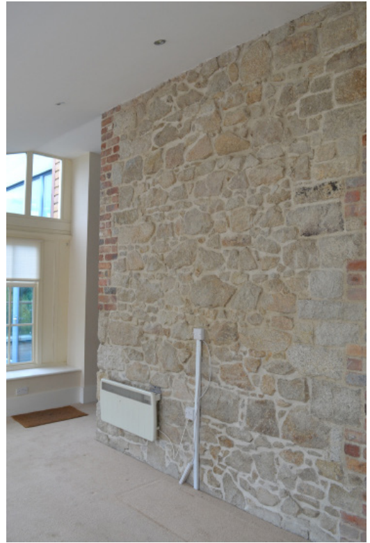
View of exposed stone rubble wall in conservatory.
