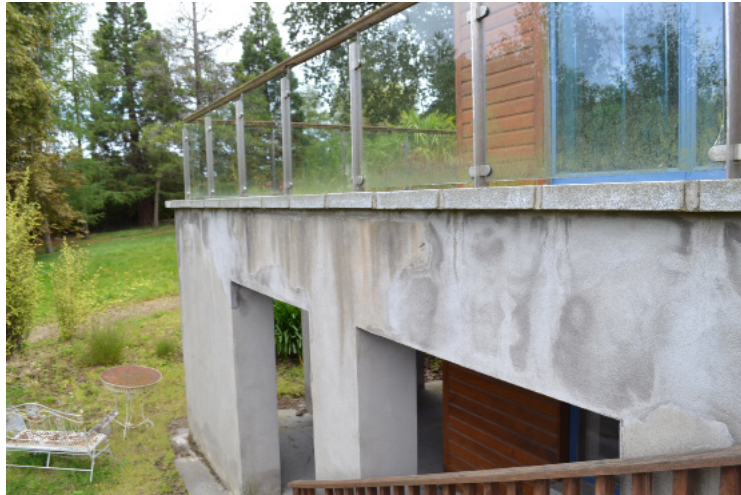
Detail of north-eastern corner of loggia/terrace.
