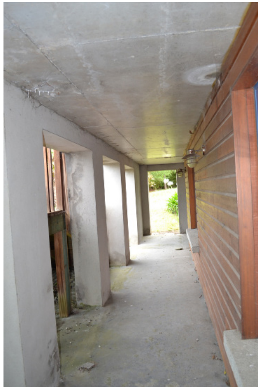
View of northern section of loggia looking to the east.
