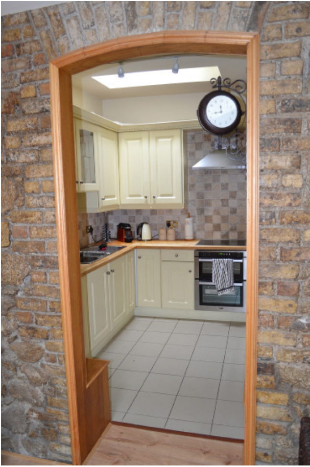
Opening in wall between extension and kitchen area.
