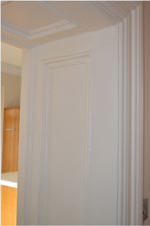
Detail of timber work on internal door to kitchen.
