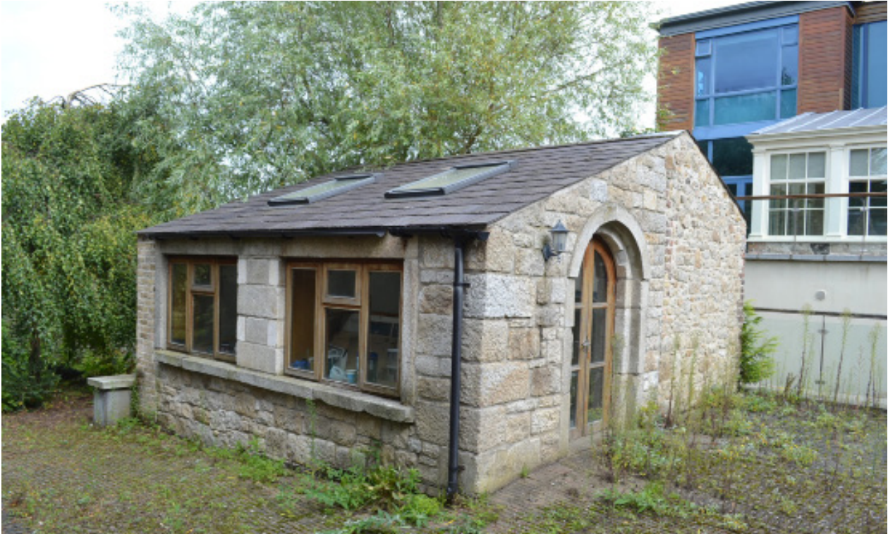
Shed as viewed from the south-west.
