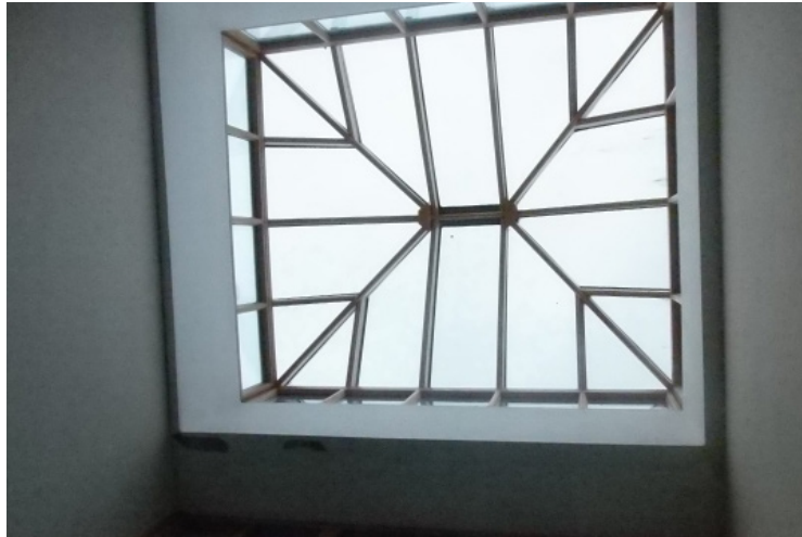
View of roof-light from staircase.
