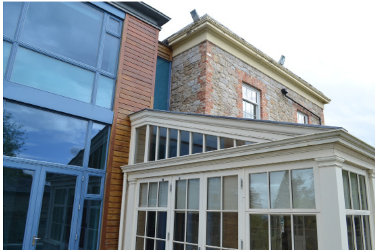
Junction between rear extension, conservatory & house.
