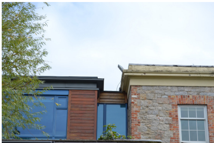
Junction between rear extension and house on west elevation.
