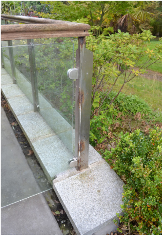
Detail of glass balustrade and concrete coping of terrace.
