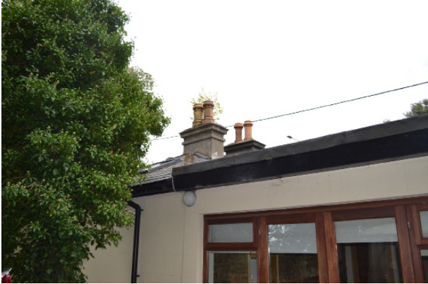
Junction between pitched rood and flat roof.
