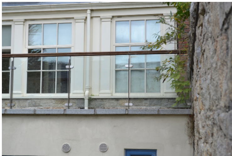
Detail of terrace guarding.
