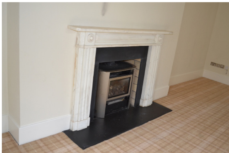
Detail of living room fireplace.
