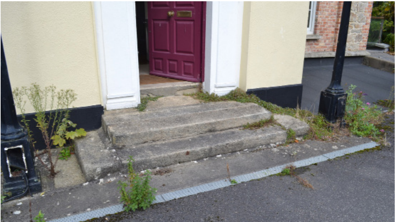
Detail of entrance lobby doors.
