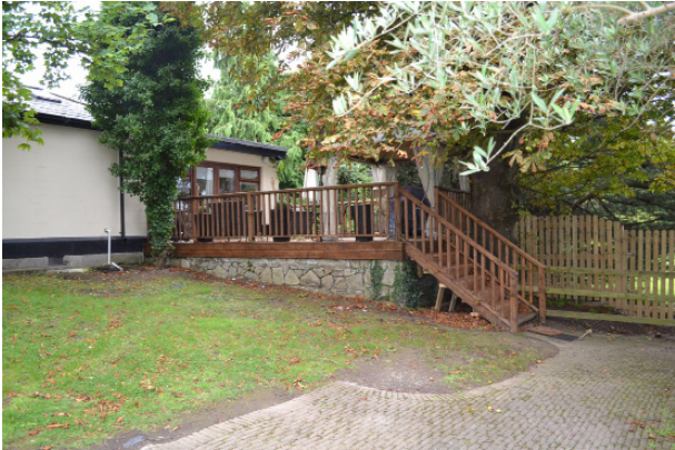
External timber terrace.
