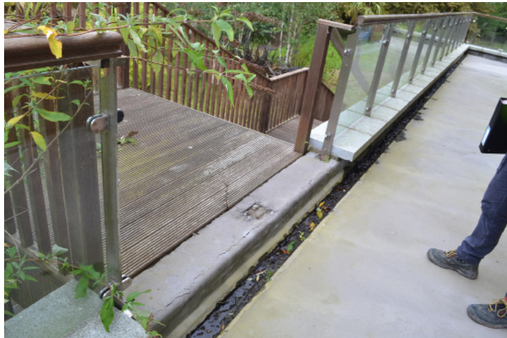
Detail of access to timber stairs from terrace.
