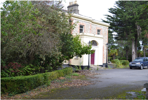
Cedar Mount - Current view from south-west.
