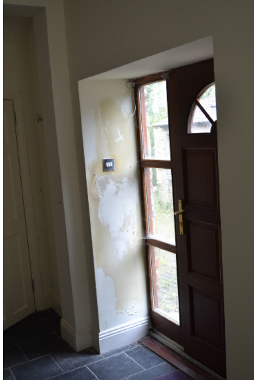
View of front door.
