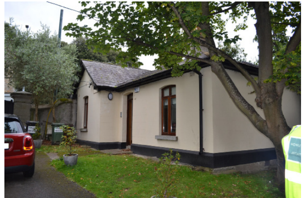
View from North East.
