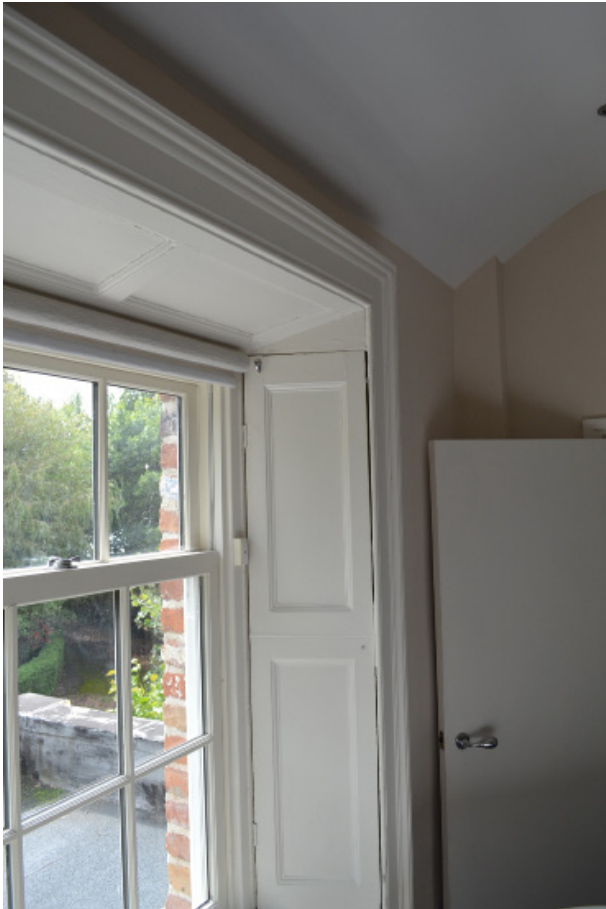
Detail of bathroom window.
