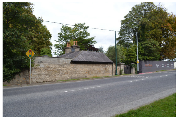
View of Stone Rubble Boundary Wall.
