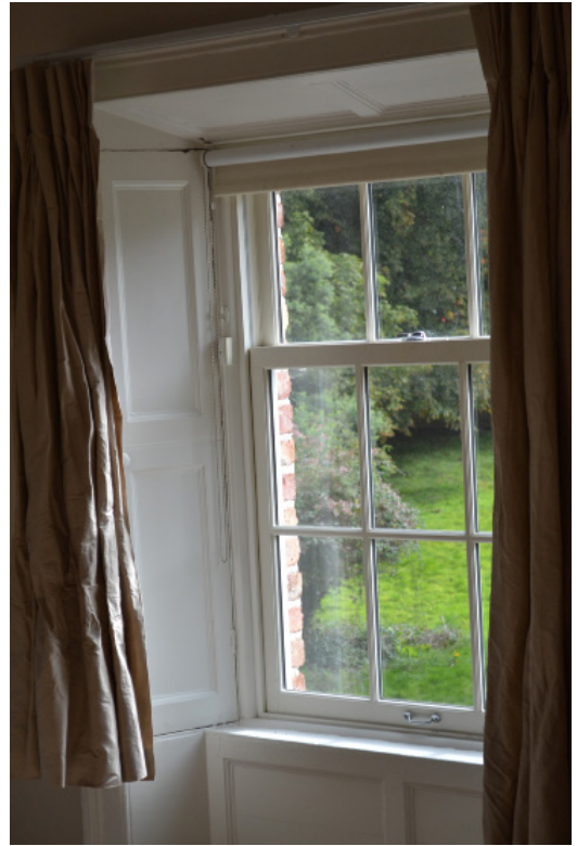
Detail of window in bedroom 02.
