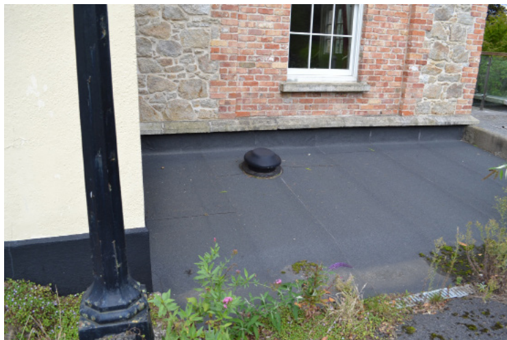
Detail of waterproofing above service space 02.
