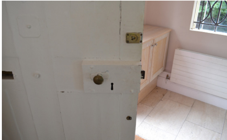
Detail of front door lock.
