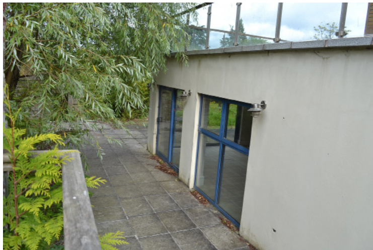
Detail of windows to North-west corner of Cedar Mount west elevation.
