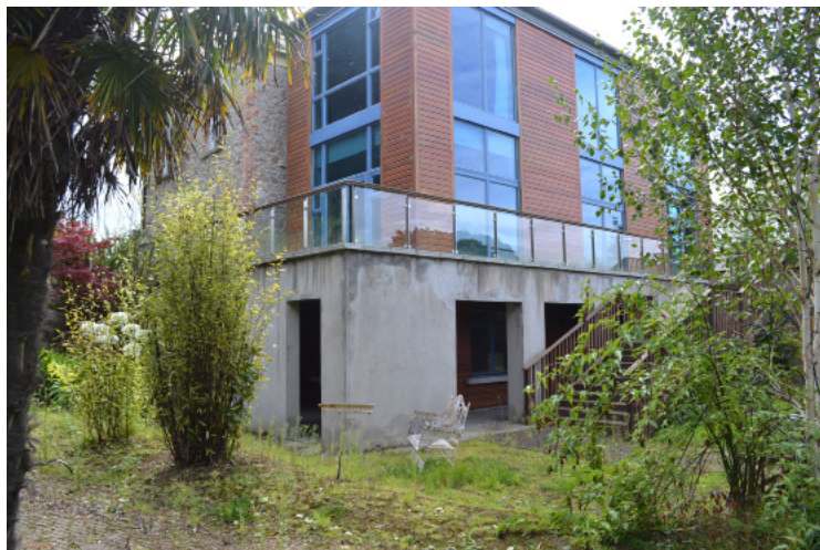
View from terrace/loggia from north-east.
