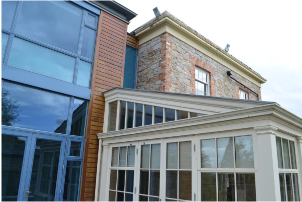
Cedar Mount - Current view of junction between rear extension conservatory and original house.
